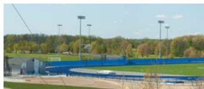
Photo Credit: GVSU The stormwater complex is sized to manage runoff from the south campus.
